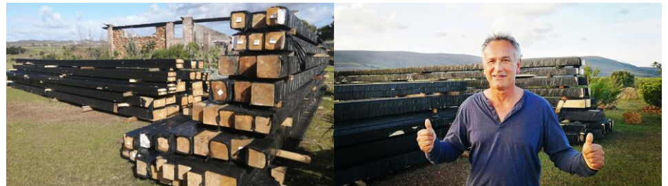
The shipment of 46m 3 Spruce beams by HWZi ( www.hwz.co.za ) arrived for the rebuild of the workshop. This is also stock for future MINI HOUSES which are set to go into production beginning 2020.
